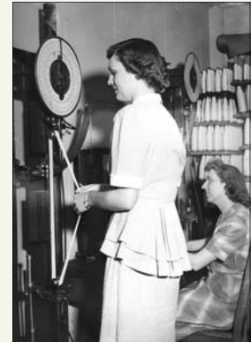
American Thread Company worker testing the strength of thread. This photo, from the Museum's archives, was scanned by students in Dr. Free's class for podcast.
