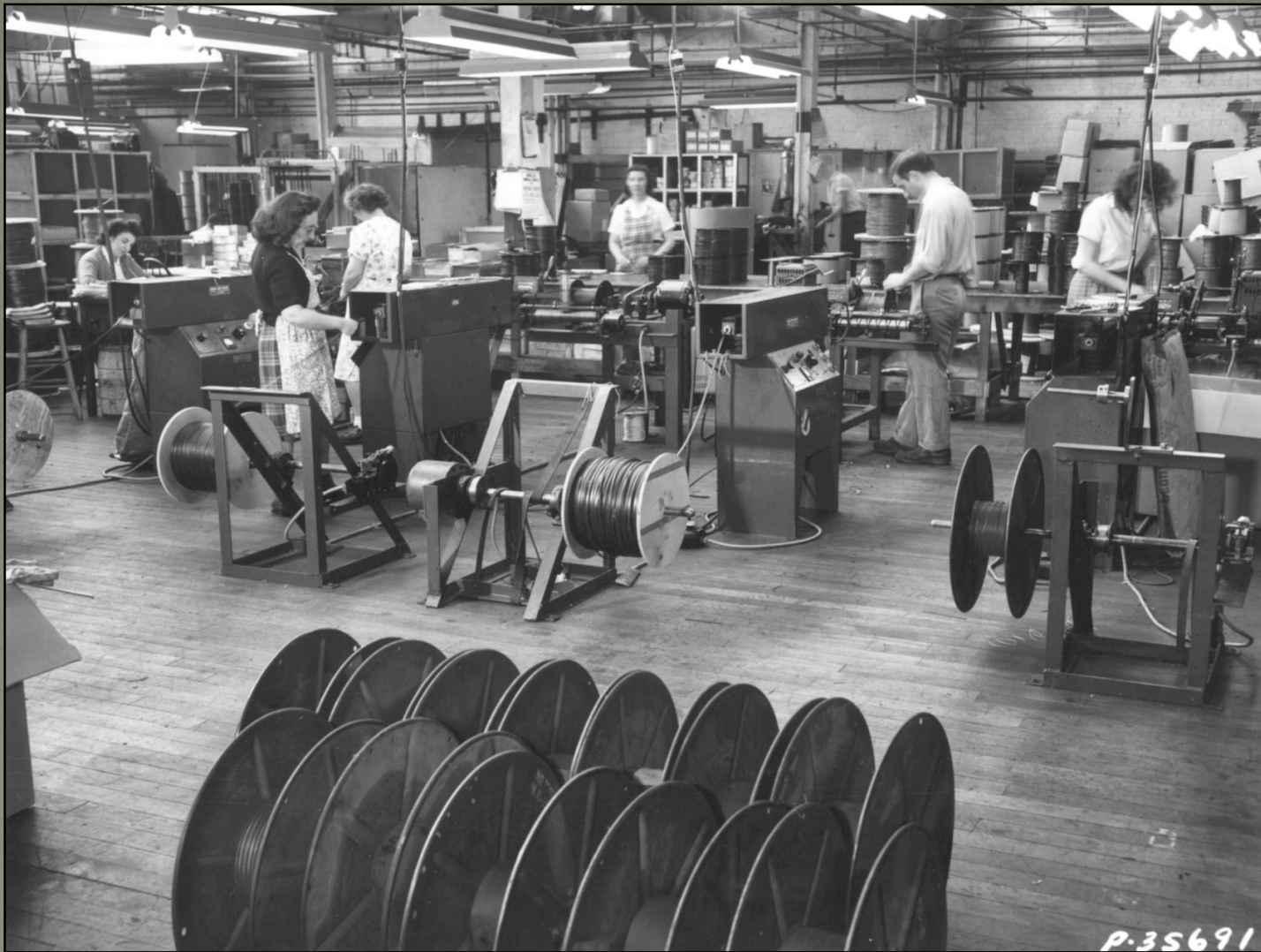
Pho-M-0526. Workers rewinding, spooling cable from large tube to shipping size, at the South Street factory of the William Brand Company, Willimantic, CT, 1949. Black and white gelatin print. Unknown photographer. From left, the workers are Bunny Lombardo, Celian Martin, unknown, Bernice Wingertman, unknown, unknown, and unknown.
