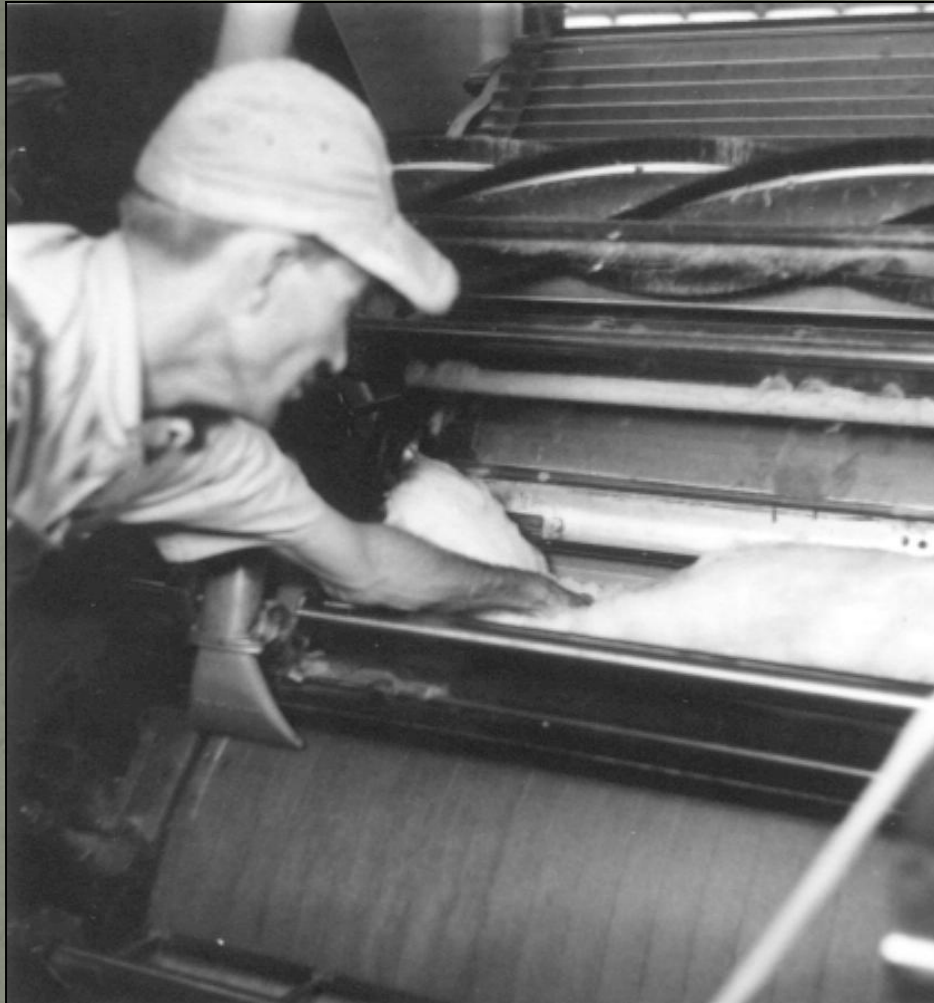
Pho-A-0674. An unidentified American Thread Company Worker demonstrates the improper use of a carding machine for a company safety brochure. Willimantic, CT, 1943. Black and white gelatin print snapshot. Unknown photographer. Carding machines were the most dangerous machines in textile mills, and unwary workers could lose fingers, hands, or even arms in industrial mishaps. What is the worker doing wrong in this photo?
