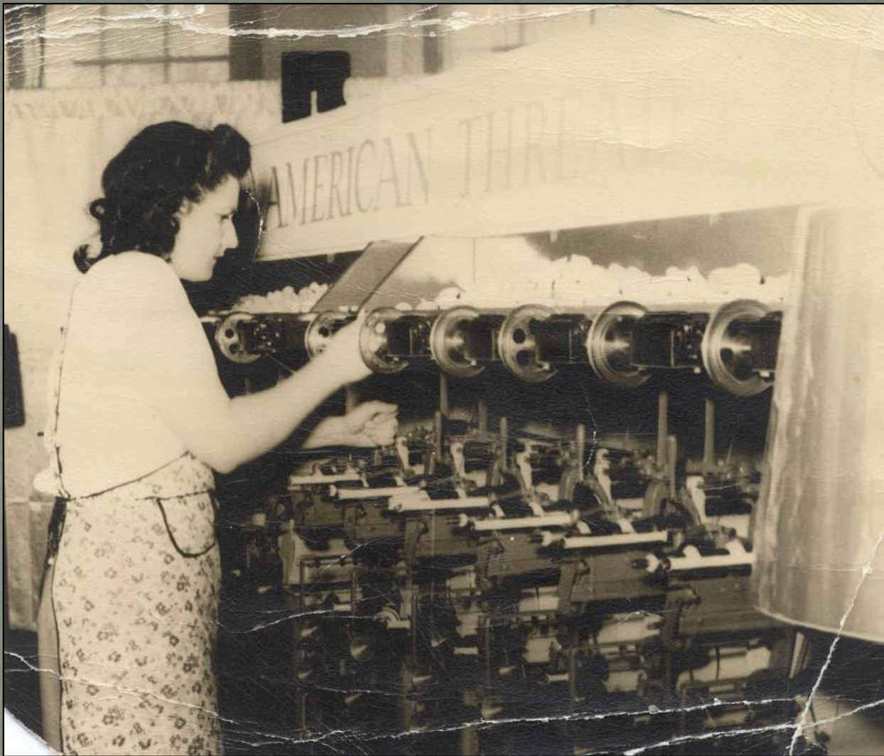
Pho-A-0599. Irene Monroe using a winder, American Thread Company, Willimantic, CT, c. 1940s. Black and white snapshot. Unknown photographer. Monroe was born in 1919, the daughter of a blacksmith. She worked at ATC for 30 years, mostly in the finishing department in Mill Number Six.
